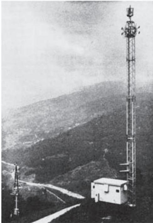
*Figure 15.6 A typical low-power television and VHF/FM rebroadcasting station*
