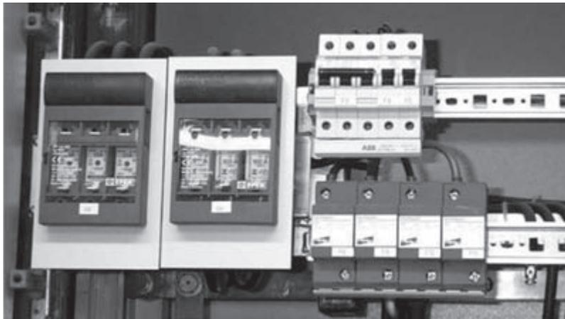
Figure 7.34 *Lightning current arrester at LPZ boundary LPZ 0<sub>A</sub>-1*
