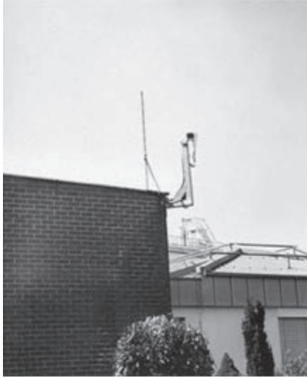
Figure 7.97 *Camera for video surveillance in the protective area of the air-termination rod*
