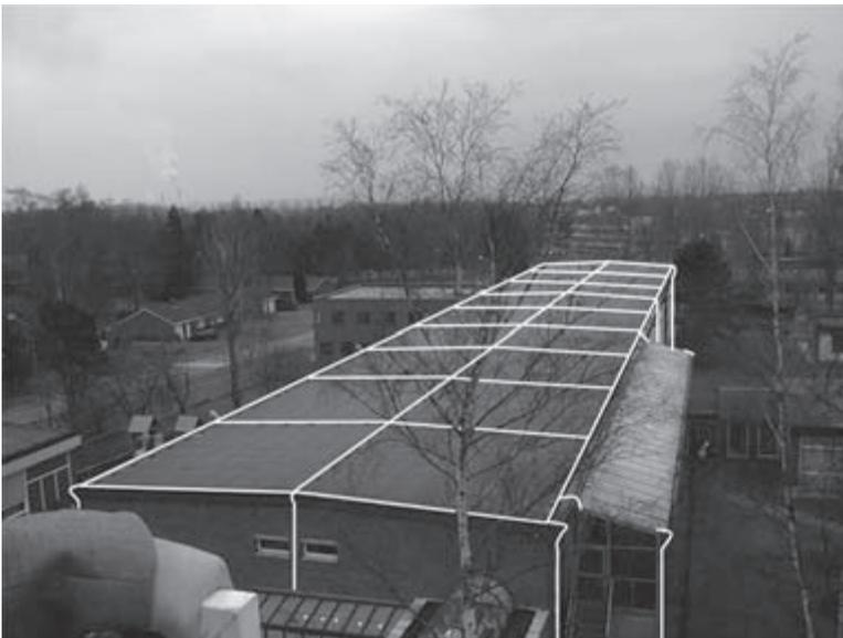
*Figure 6.4 Flat roof protected according to the mesh method*
