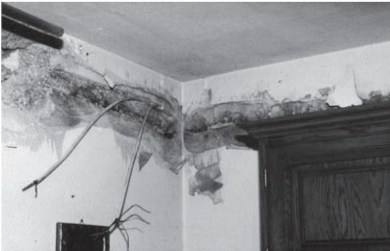
*Figure 7.6 Punctures to concealed cables due to lightning strike*
