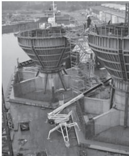
Figure 14.23 Concrete offshore foundations under construction on a barge for later deployment at offshore (photo by the author)
