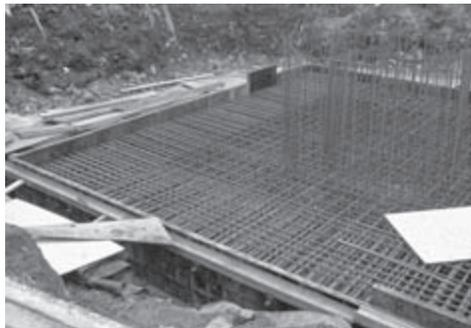
*Figure 14.11 Steel reinforcement of a foundation for a 1 MW wind turbine. The dimensions of the horizontal plate  $L \times W \times H$  are  $\sim 10 \text{ m} \times 10 \text{ m} \times 1 \text{ m}$  (photo by the author).*
