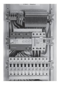
Figure 7.63 Series connection with a busbar
