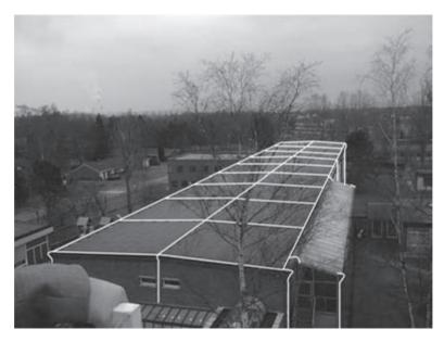
Figure 6.4 Flat roof protected according to the mesh method
