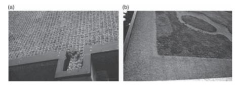
Figure 7.15 (a) Galvanized construction steel shielding roofs. (b) Use of galvanized construction steel mats for shielding, for example in the case of planted roofs.
