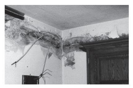
Figure 7.6 Punctures to concealed cables due to lightning strike
