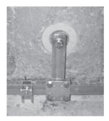
*Figure 7.24 Connection of the ring equipotential bonding bar with the equipotential bonding network via a fixed earthing point*
