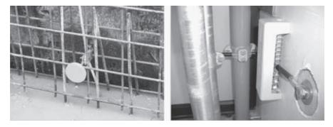
Figure 7.27 Installation of fixed earthing point
