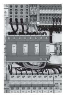
*Figure 7.42 Combined lightning current and surge arrester: DEHNventil modular*<sup>®</sup> *TNS*
