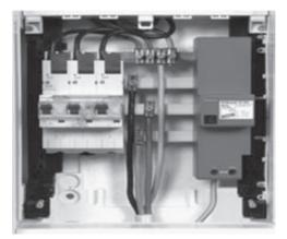
Figure 7.12 DEHNventil ZP lightning current arrester installed in a busbar terminal field of a meter installation
