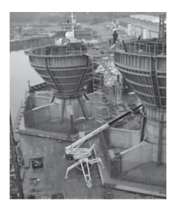
*Figure 14.23* Concrete offshore foundations under construction on a barge for later deployment at offshore (photo by the author)
