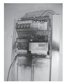
Figure 7.7 A distribution panel damaged by lightning strike
