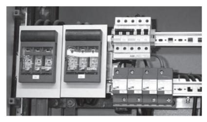
Figure 7.34 Lightning current arrester at LPZ boundary LPZ  $0_A$ -1
