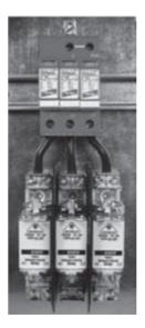
Figure 7.87 Application of DEHNguard surge arrester, DG TNC FM,  $U_c = 750 V$
